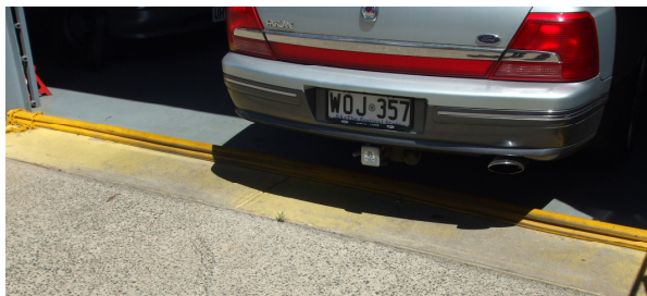
Bunding the workshop entrance can be a good solution. The yellow rubber strip is bunding.
